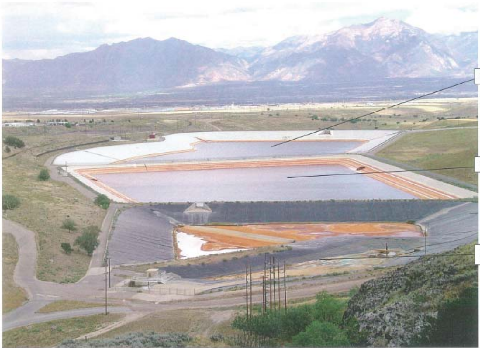
Large Reservoir at Bingham Creek. View: East
